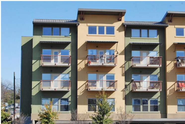
Facade modulation provided by vertical shifts and balconies.
