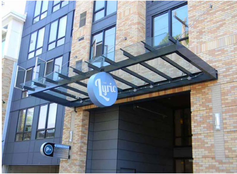
Building lobby with canopy to give the entry prominence.
